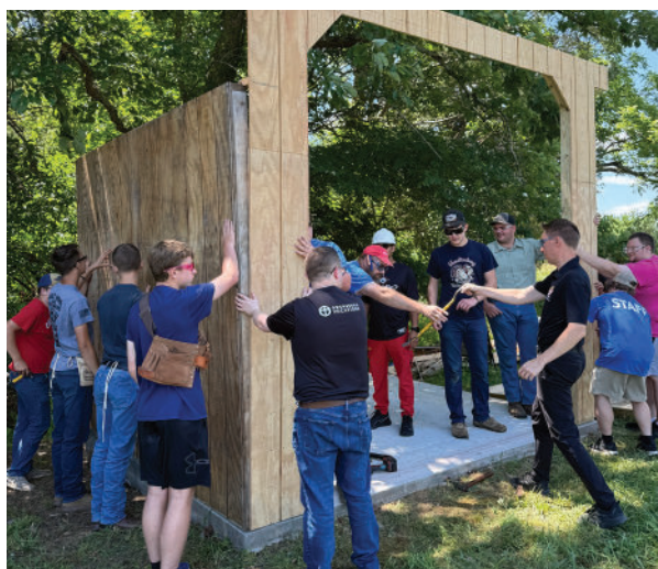
COURTESY OF FR. COREY D. BRUNS Participants of the Office of Vocations' Quo Vadis Camp during June 14-17 help build a storage/maintenance shed.
