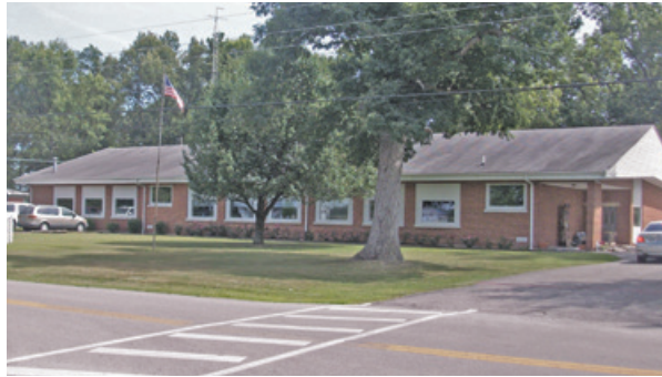
The school building today displays new windows, a new front door, drop ceilings and a fenced-in playground for St. Paul preschoolers. Photo courtesy of St. Paul School.
